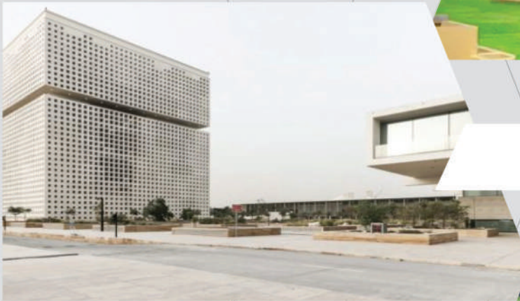
Qatar Foundation Headquarters Building & Strategic Studies Center
